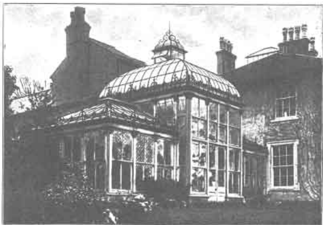
No. 2.—CONSERVATORY erected for A. J. New, Esq., Ruddington, Notts.
