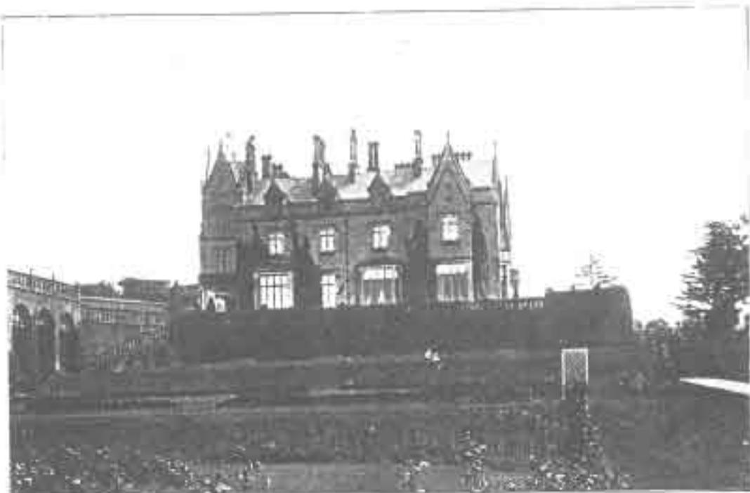
Lilleshall House, Newport, Salop. Heated by Hot Water for His Grace the Duke of Sutherland.
